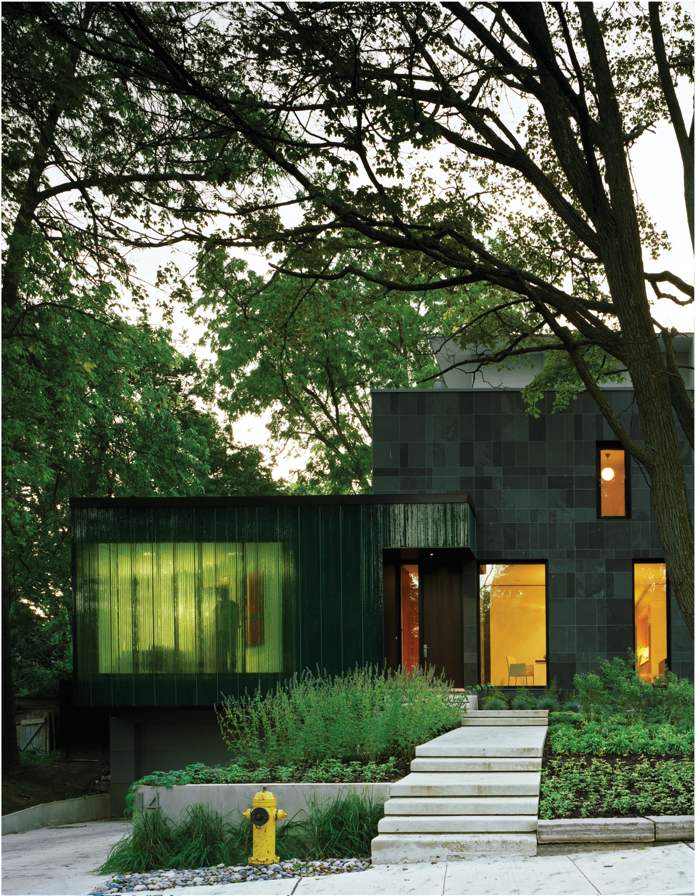
Emerald in the rough The elegant front facade features a four-metre-high shimmering screen of green glass set against a charcoal slate background.
